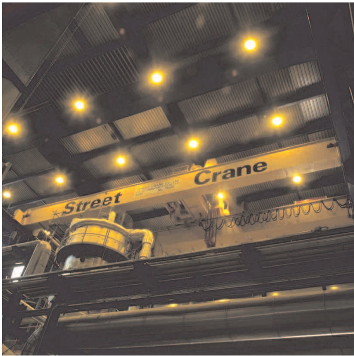
85t Turbine Handling Crane A.B.B. Power Generation
