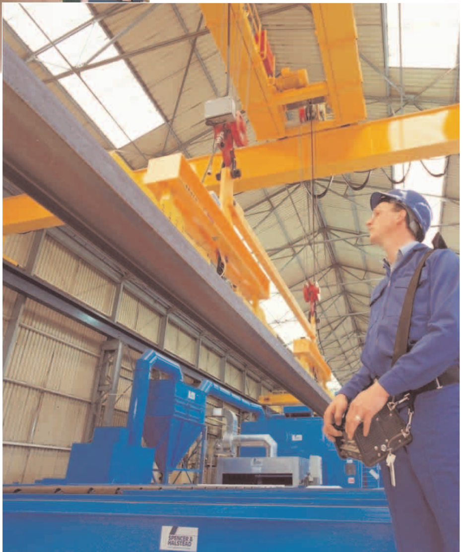
15t Twin Hook Magnet Crane British Steel
