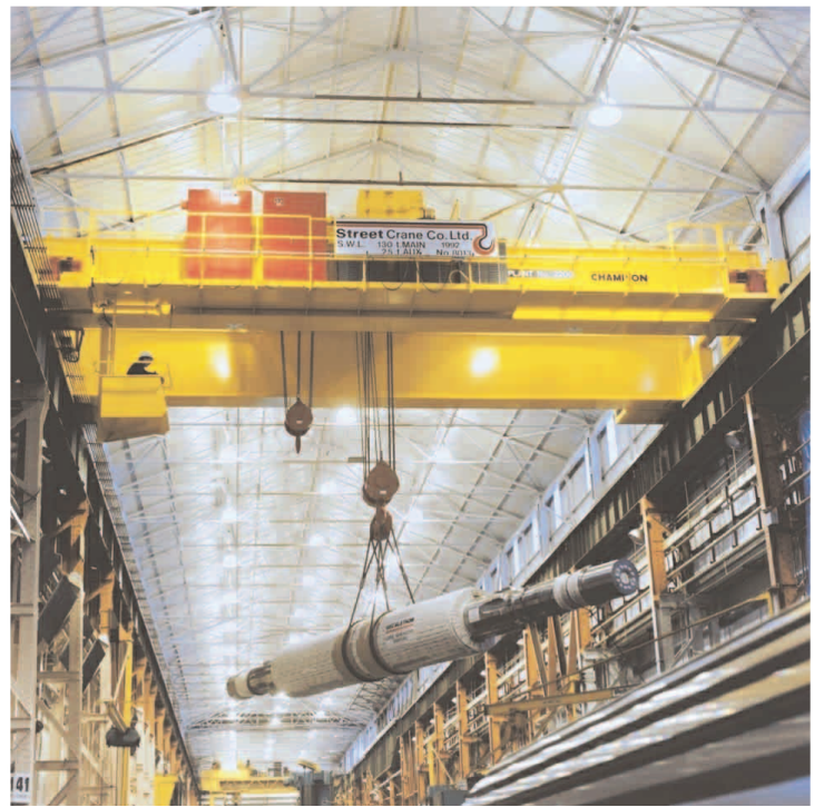
130t Turbine Handling Crane G.E.C. Alstom
