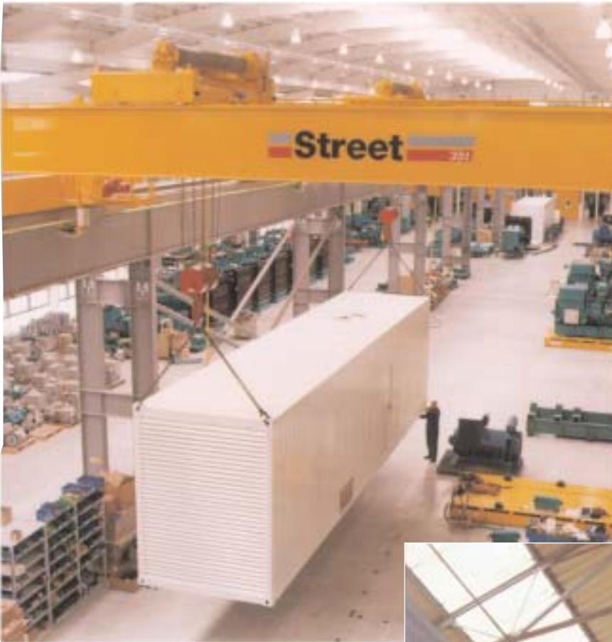
2 No. 35t Tandem Lift Cranes Cummins Power Generation
