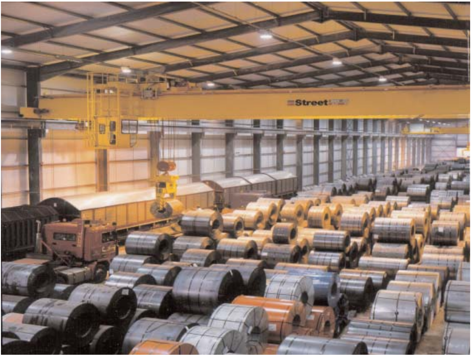
35t Main Hoist / 5t Auxiliary Hoist Coil Handling Moss Construction
